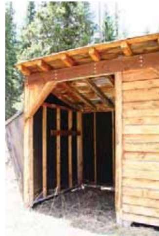
Figure 6: Roof Framing at Ridge
