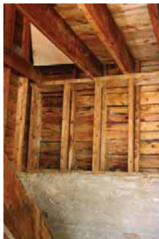
Figure 32: Floor Joist Support at Back
