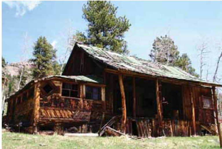
Figure 12: Exterior View of Staunton House
