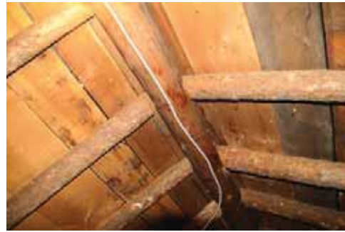
Figure 3: Roof Framing at Ridge
