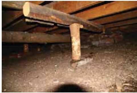
Figure 2: Floor Framing
