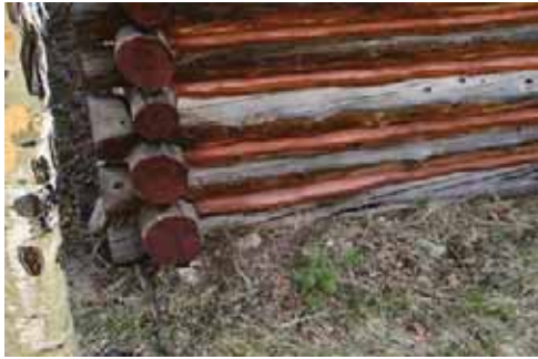
Figure 10: Corner Joint
