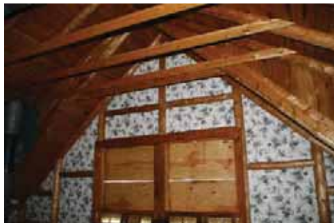
Figure 20: Roof and Gable End Wall Framing
