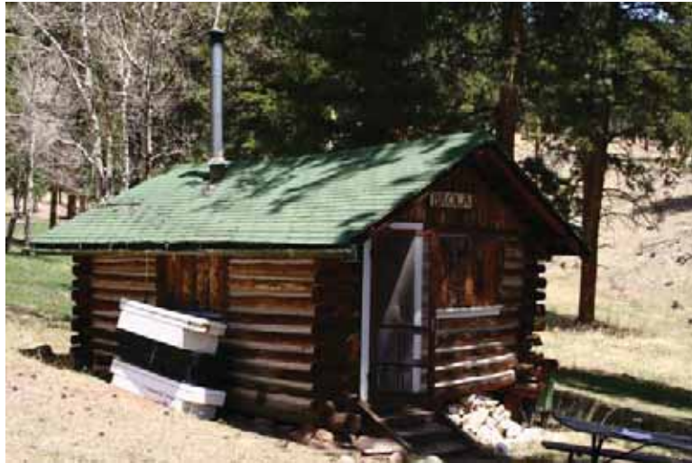
Figure 17: Exterior View of Brola Cabin
