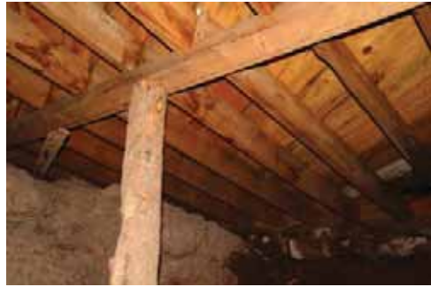
Figure 29: Floor Framing in Cellar
