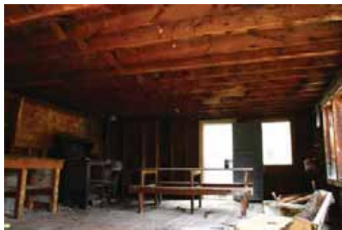
Figure 30: First Level with Upper Floor Framing
