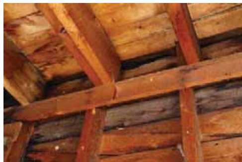
Figure 31: Floor Joist Support at Front
