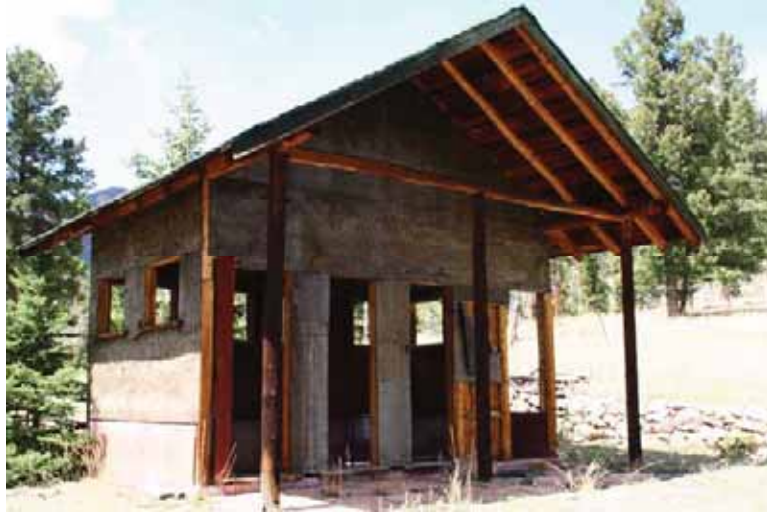
Figure 22: Exterior View of Bath House
