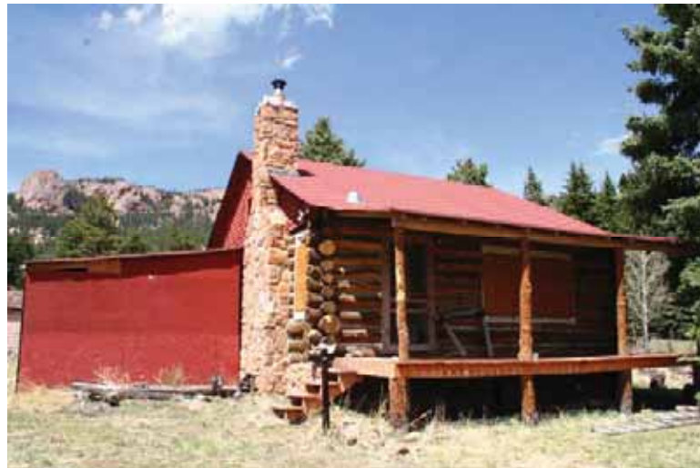
Figure 24: Exterior View of Large Cabin
