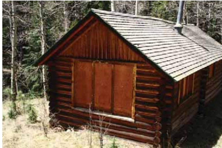
Figure 9: Exterior View of Small Cabin
