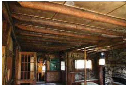
Figure 14: Loft/Roof Framing
