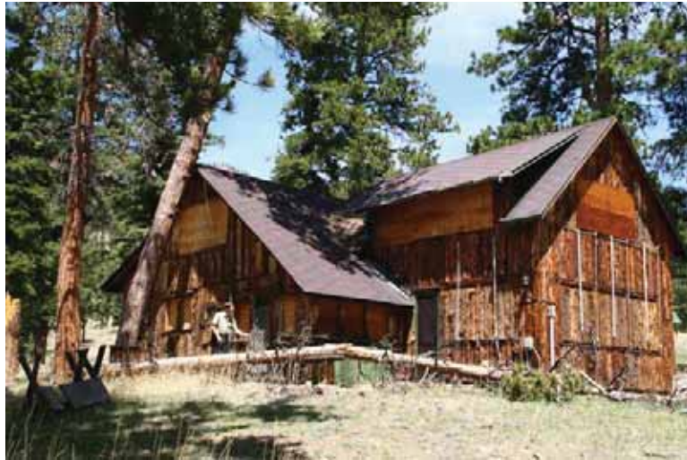
Figure 19: Exterior View of Richardson Cabin
