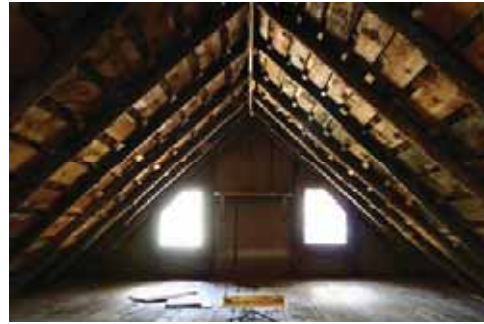
Figure 16: Roof Framing at Ridge
