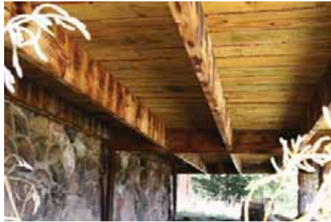
Figure 25: Porch Floor Framing
